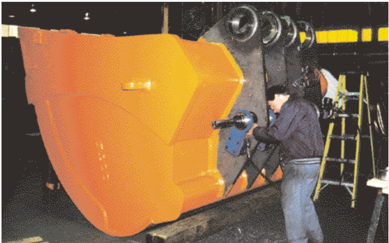
The BB 5000 boring bar from Climax Portable Machine Tools is set up to line-bore the pin bosses on this 14-cubic-yard bucket.
